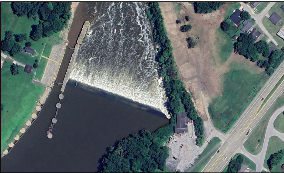
Figure 1: Final site selection aerial view
